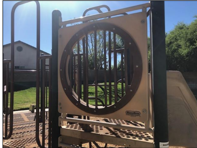
Play Equip repairs at Sagecrest Park
